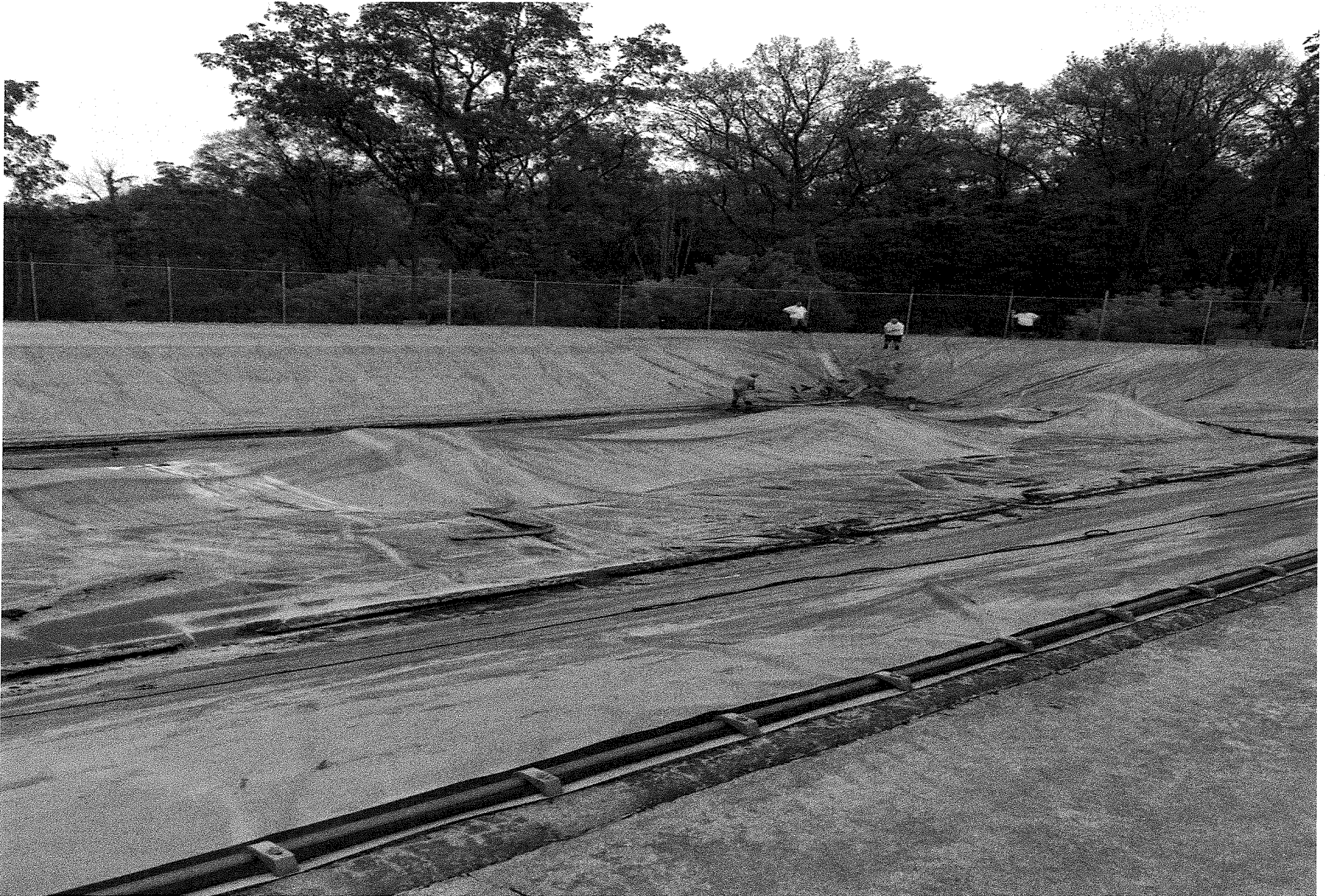
Dale Street Reservoir Cover
